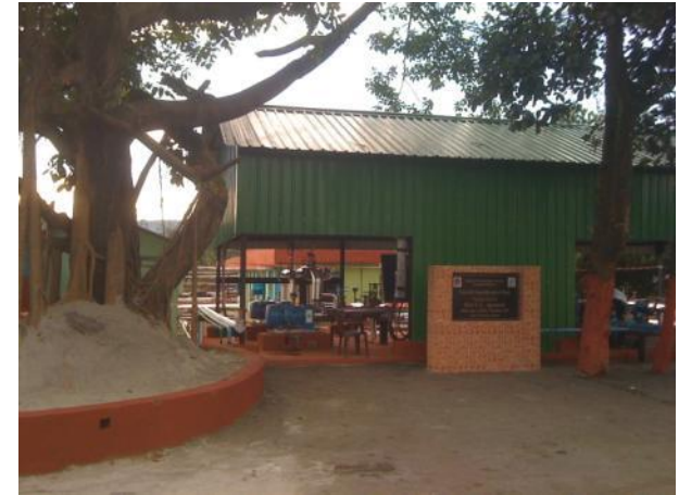
Entrance to Emulsification Plant
